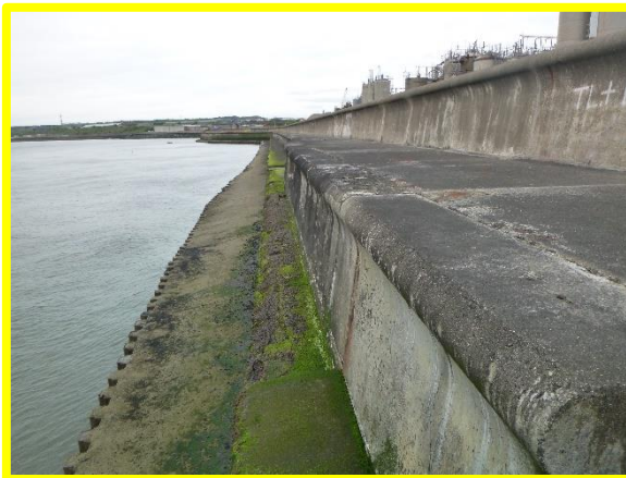
North end of Spur Barrier upper wall. (Asset Ref. No. 121AB901B0802C04)
