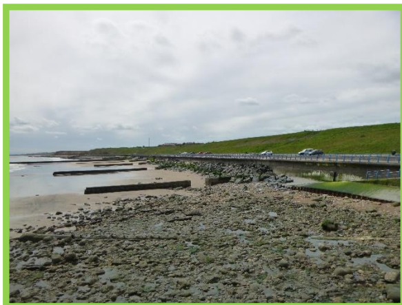
Hendon Seawall, groynes and rock armour (Asset Ref. No. 121AB901B0803C02)
