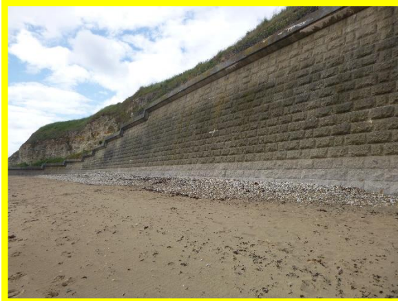
Masonry wall generally in good condition (Asset Ref. No. 121AB901B0605C01)
