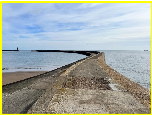
New South Pier, upper deck. (Asset Ref. No. 121AB901B0703C01)
