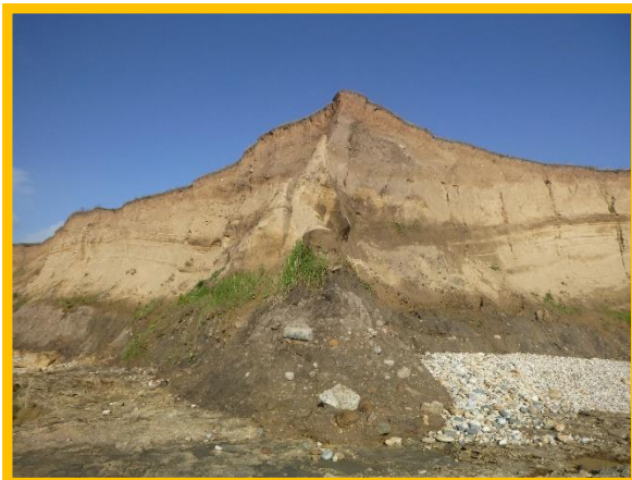
Recent Slumping along Halliwell Banks (Asset Ref. No. 121AB901B0804C02)
