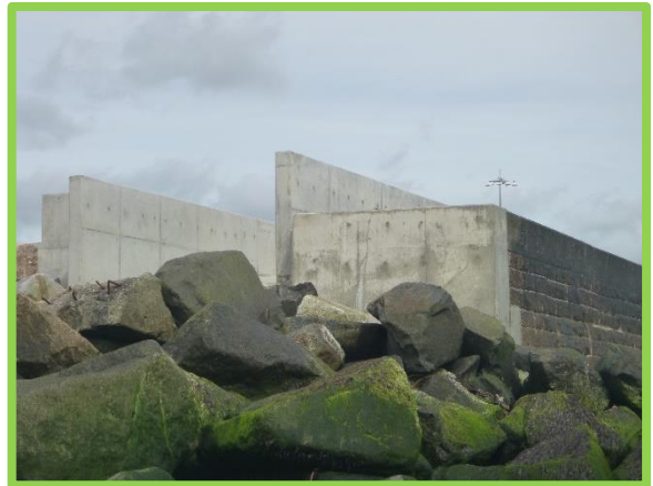
Southern end of wall repaired. (Asset Ref. No. B901B0801C03)
