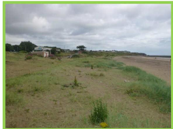
View towards north boundary, shingle berm at toe. (Asset Ref No. 121AB901B0602C01)
