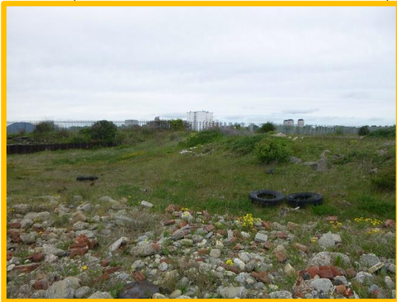
Informal transition between infill (C08) and sheet pile wall (C07). (Asset Ref. No. 121AB901B0802C07).
