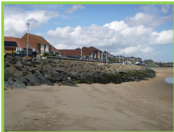
Even profile and crest level on rock armour revetment . (Asset Ref. No. 121AB901B0702C02)
