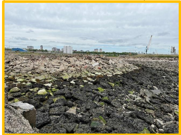
South side of basin taken from South West Breakwater. (Asset Ref. No. 121B901B02C06)
