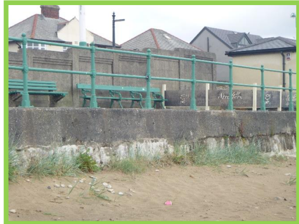
Original coping in fair condition. (Asset Ref No. 121AB901B0603C01)
