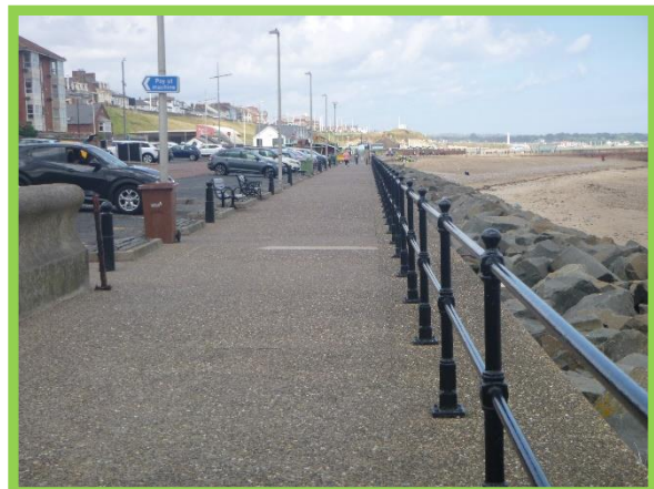
Rock armour and promenade in good condition. (Asset Ref. No. 121AB901B0702C02)
