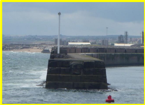
Northern tip of New South Pier. (Asset Ref. No. 121AB901B0703C01)
