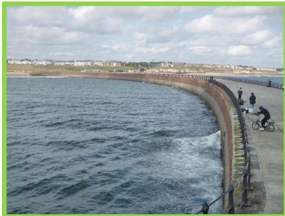
Recently replaced handrail and coping blocks. (Asset Ref. No. 121AB901B0702C04)
