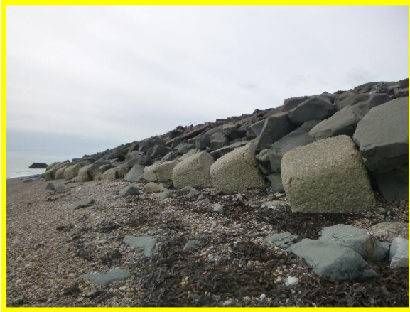
Rock/rubble revetment north of derelict groyne. (Asset Ref. No.121AB901B0801C02)
