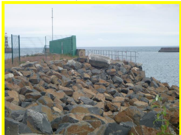
Former breach infilled with rock armour and grout. (Asset Ref. No. 121AB901B0702C03)
