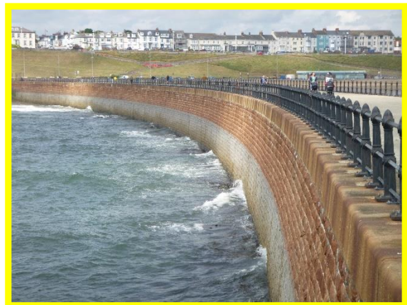
Roker Pier northern (inner) face (Asset Ref. No. 121AB901B0702C04)
