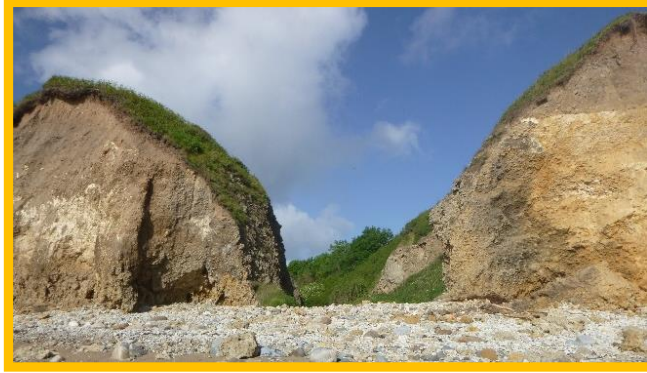
Southern boundary of frontage at Ryhope Dene (Asset Ref. No. 121AB901B0804C02)
