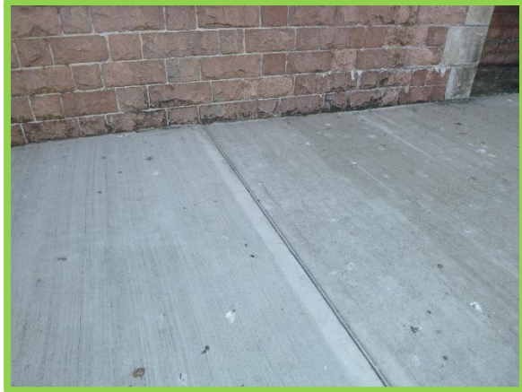
Repaired slabs in good condition. (Asset Ref. No. 121AB901B0703C01)
