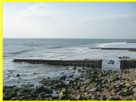
Concrete groyne, beach levels similar to 2020. (Asset Ref. No. 121AB901B0803C02)
