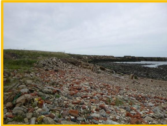
Tipped rubble at northern end of South Outlet basin. (Asset Ref. No. 121AB901B0801C08)
