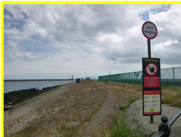
Vegetation growth on haulage path built for delivery of rock repairs. (Asset Ref. No. 121AB901B0702C03)
