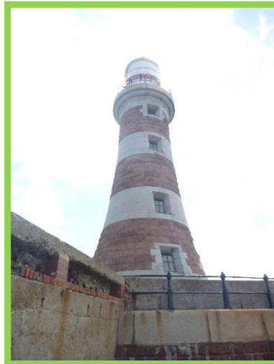
Recently refurbished lighthouse. (Asset Ref. No. 121AB901B0702C04)
