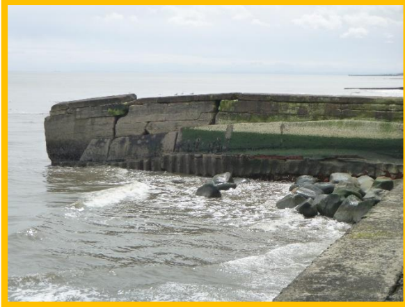
Breakwater with nose detached, from north side. (Asset Ref. No. 121AB901B0803C02.)
