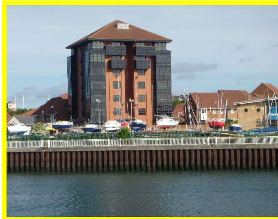
Sheet piling along southern face of wall (Asset Ref. No. 121AB901B0702C03)
