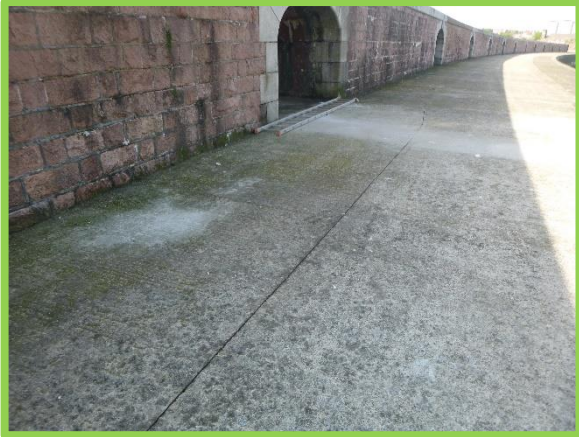
Contraction joint has been cut into slabs. (Asset Ref. No. 121AB901B0703C01)
