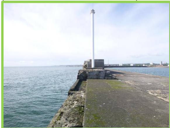
Recently installed navigation light column. (Asset Ref. No. 121AB901B0703C01)
