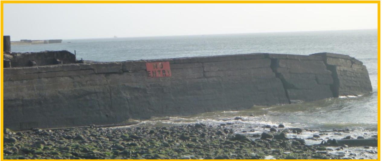
Breakwater with nose detached, from south side.(Asset Ref. No. 121AB901B0803C02)
