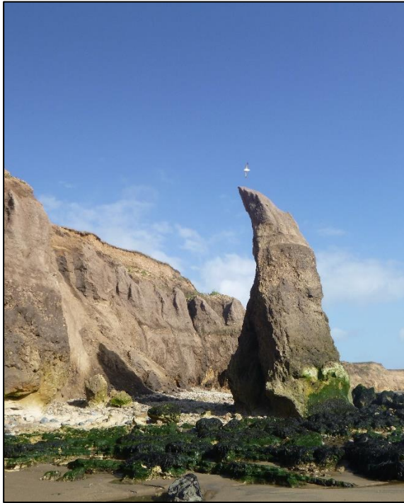
Sea stack near Ryhope Village Dene (Asset Ref. No. 121AB901B0804C02)
