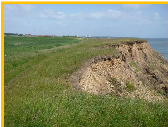
Recent slumping at Salterfen Rocks (Asset Ref. No. 121AB901B0804C03)
