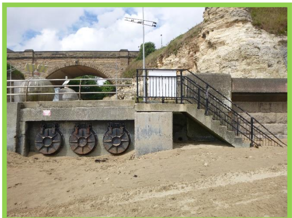
Outfall pipes at north end of Marine Walk. (Asset Ref. No. 121AB901B0605C02)
