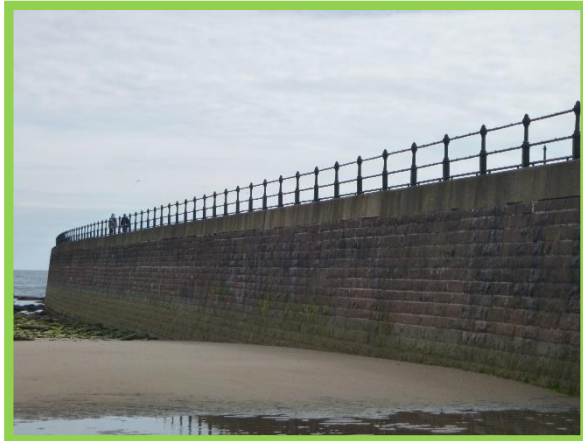
Northern (outer) face of pier (Asset Ref. No. 121AB901B0702C04)
