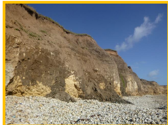
Recent large slump south of Pincushion (Asset Ref. No. 121AB901B0804C02)
