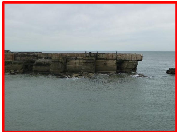
North East Pier viewed from south. (Asset Ref. No. 121B901B0801C04)
