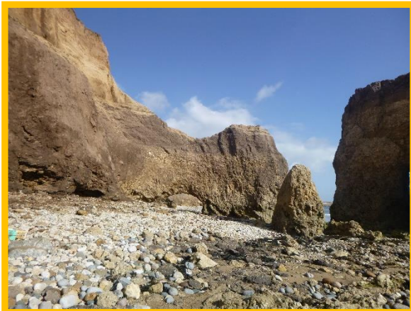
Slumping and seepage near sea stack at Pincushion (Asset Ref. 121AB901B0804C02)
