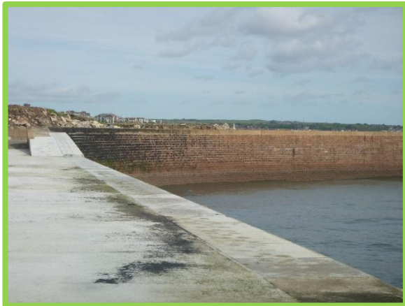
New precast coping stones. (Asset Ref. No. B901B0801C03)
